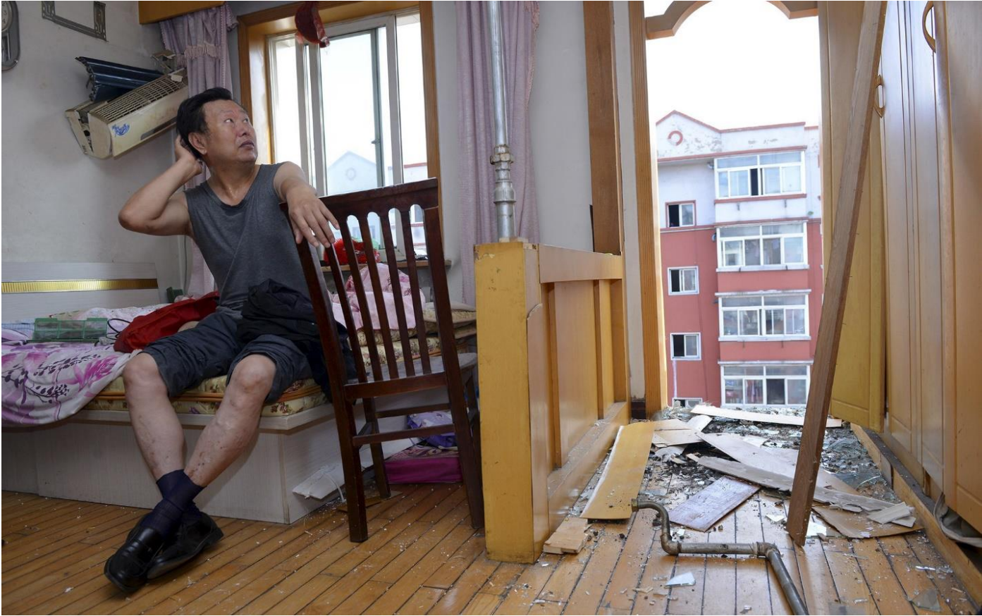
Man looks at balcony that fell off of 13 year old apartment.
