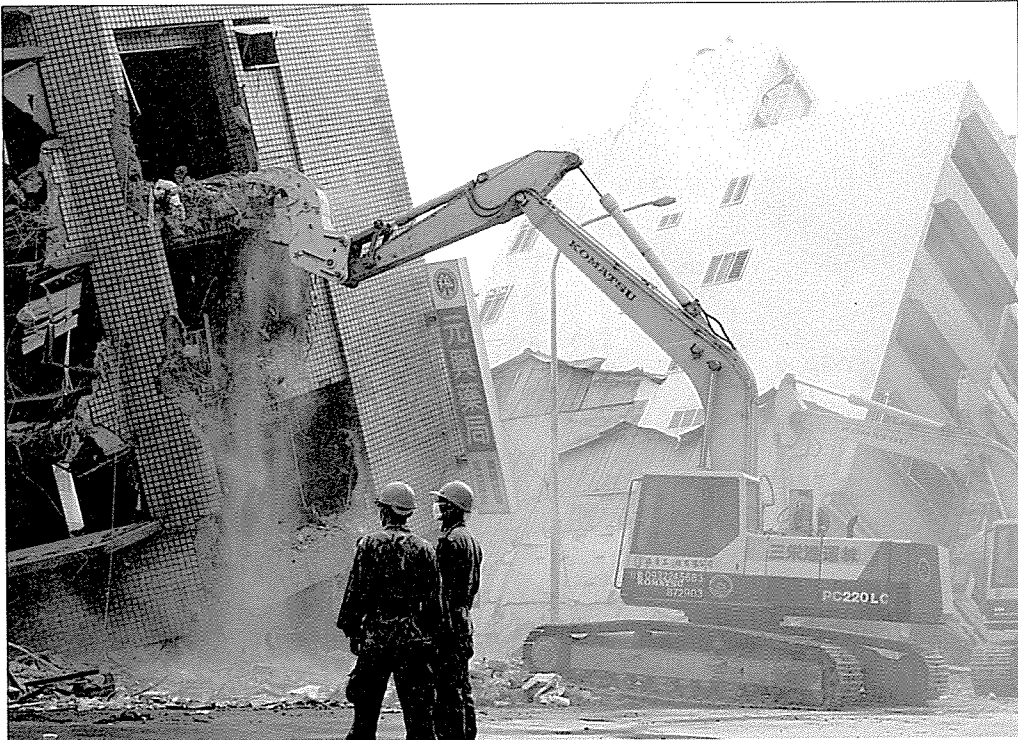
ROC Armed Forces assist in “921 Devastating Earthquake” Rescue—to dismantle dangerous buildings.
