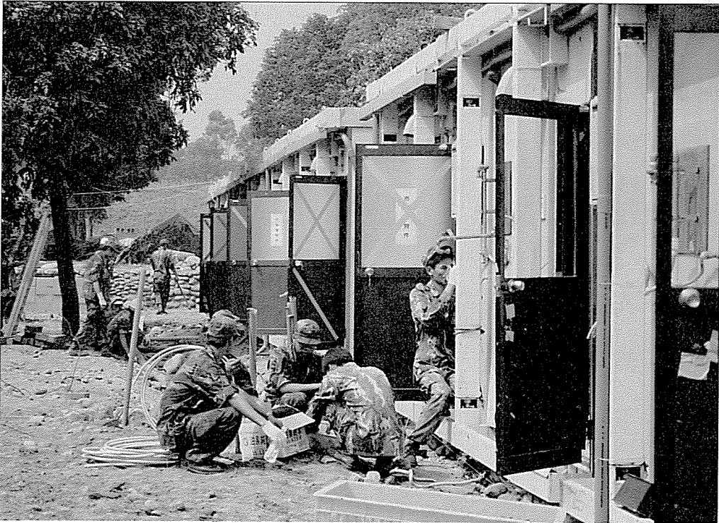
ROC Armed Forces assist in “921 Devastating Earthquake” Rescue—to construct temporary combination houses.
