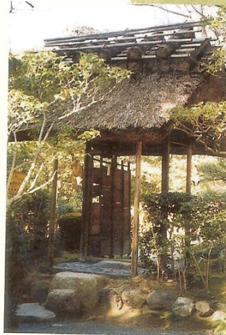
The Kayamon Gate is constructed of poles covered with a grass roof. On top of the roof is a bamboo and log frame designed to help hold the grass in place.
